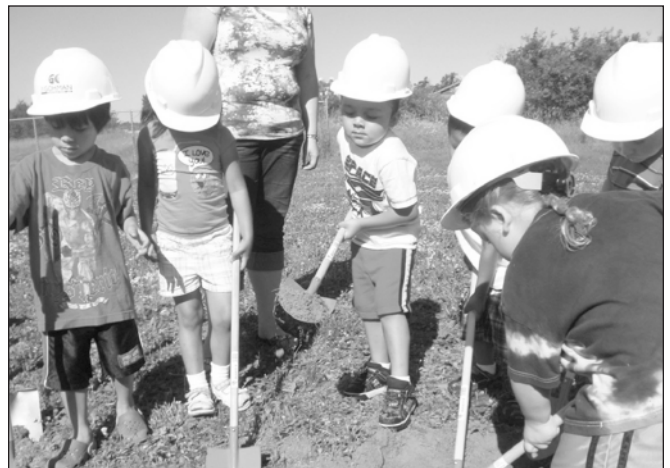
Mille Lacs Band Head Start and Early Head Start students helped break ground on the Band's new early education building in District I. The building is scheduled to be complete in August 2012.
